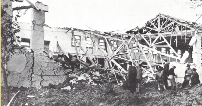
November 1944 bomb damage
